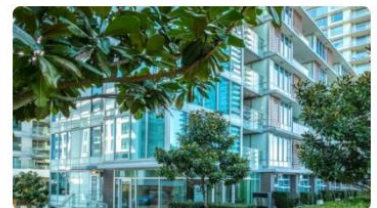
GEC Marine Gateway – South Tower
