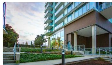
GEC Marine Gateway – North Tower
