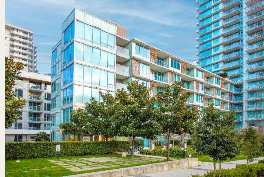
GEC Marine Gateway North Tower
