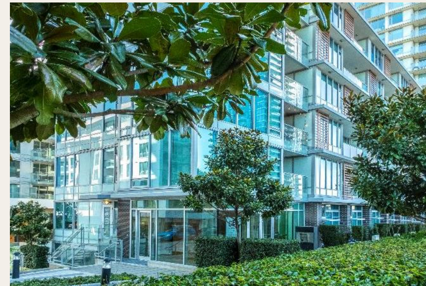
GEC Marine Gateway South Tower
