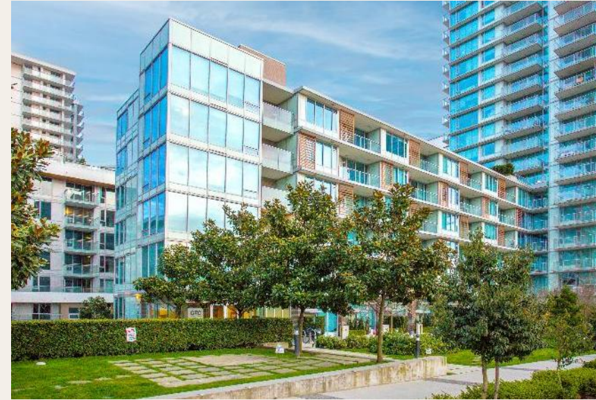
GEC Marine Gateway North Tower
