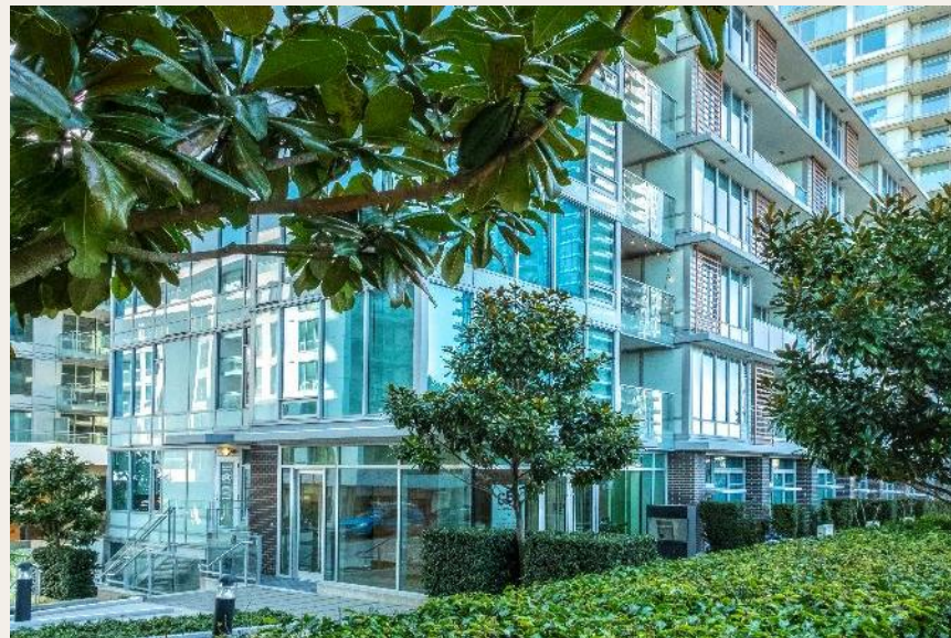
GEC Marine Gateway South Tower
