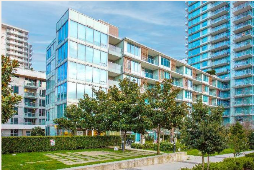
GEC Marine Gateway North Tower
