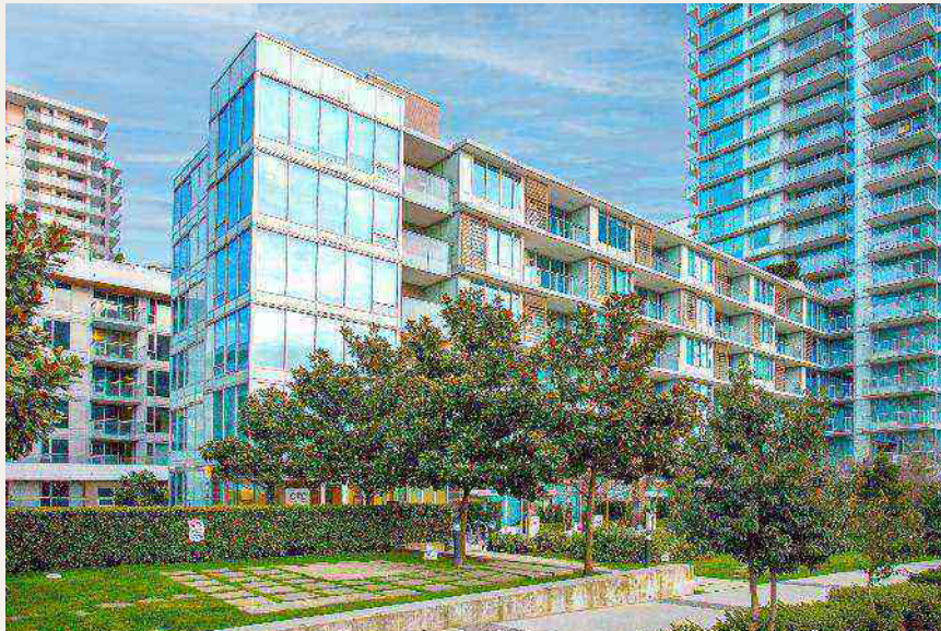
GEC Marine Gateway North Tower
